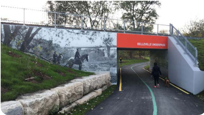
Belleville Underpass – Lower Don Trail, Toronto, ON
